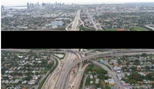
95 Express Phase 1B construction at I-95/SR 112 interchange.
